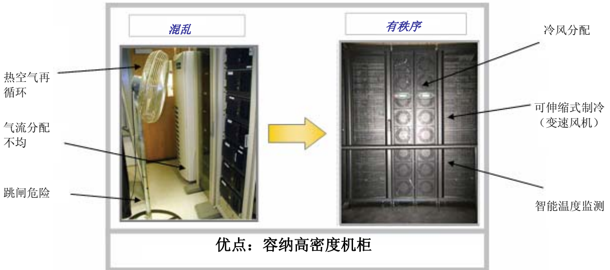
图6 – 转至 contained close-coupled™ （密闭紧耦合式）制冷
